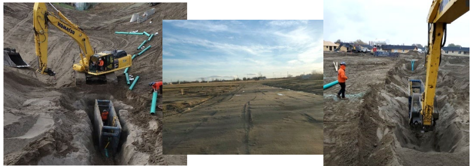
21-033 River Ridge Estates: Rock and paving left
