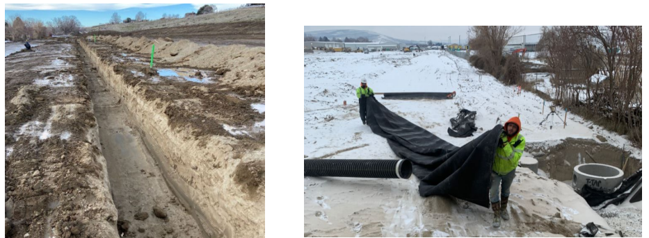
21-016 Dale Avenue: Rock and paving left
